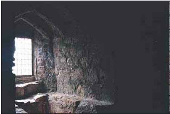
A window antechamber in the thickness of the wall still lets in a lot of light.
