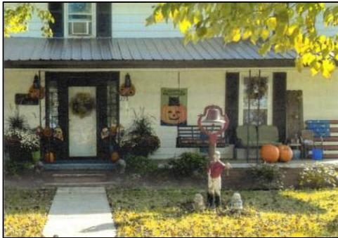
glass on both sides of the front door is single pane. It has no insulation value. The glass was made back in 1860, and it has a blue tint. I assume because it was made with a mixture of lead. I replaced all of the other windows in the two story house. But I kept the windows on both sides of the front door. I had storm windows crafted and installed in front of the two windows. I had Plexiglas installed on the inside of the glass, in the foyer. This created a dead-air space that
