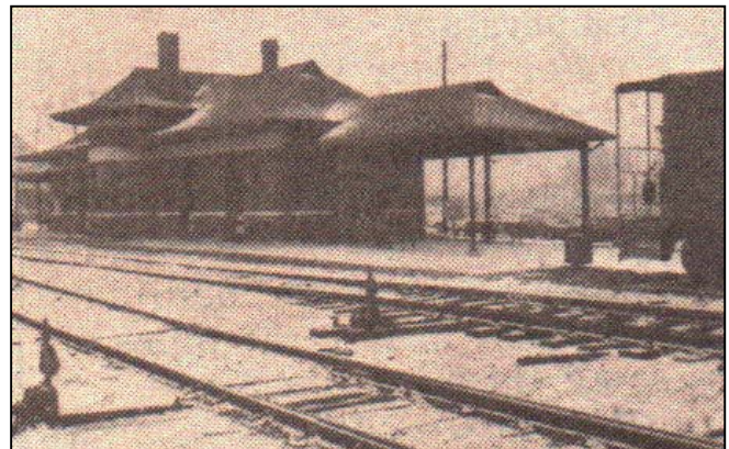
The Cookeville Depot was built in 1909. This Victorian building was constructed of brick and was very unusual for the area.
