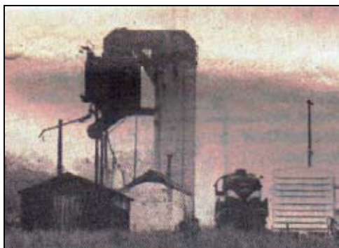
The coal chute and sand house as it appeared in Monterey, 1966. Today the tall block structure is all that remains.
