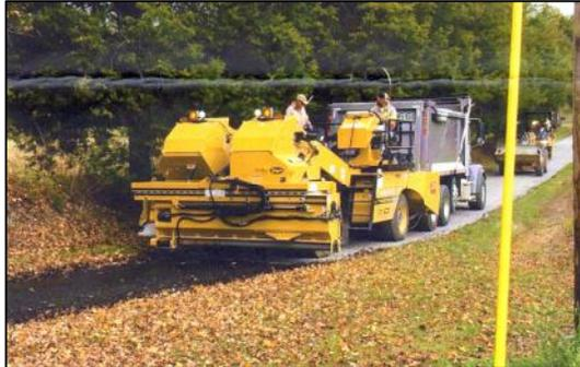
the aggregate chips that had just been graded. I was at the top of the hill and I noticed some autumn leaves, from a nearby maple tree, fall on top of the liquid asphalt. They became entombed in the liquid asphalt. Within a minute, the chip spreader followed the asphalt distributor truck and put down a second chip application. This was followed by a rubber-tire roller that sets the chips into the liquid asphalt. It takes two to four passes
