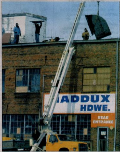
Workers use a crane to remove a vent during the ongoing renovations of the old Maddux Hardware building on Cookeville's Courthouse Square Wednesday.
