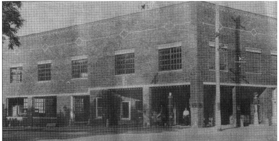
The building was the Diamond Service Station in the 1920's.
