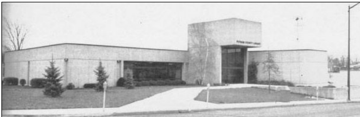
Putnam County's new modern library, located on East Broad Street across from City Hall. Cookeville, TN
